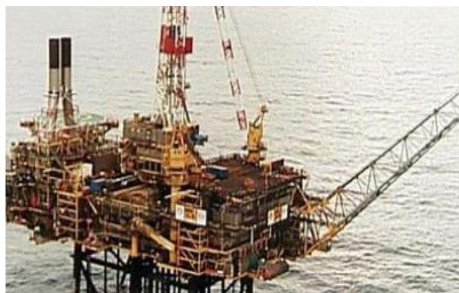
Shell's Gannet platform off the Aberdeenshire coast.
